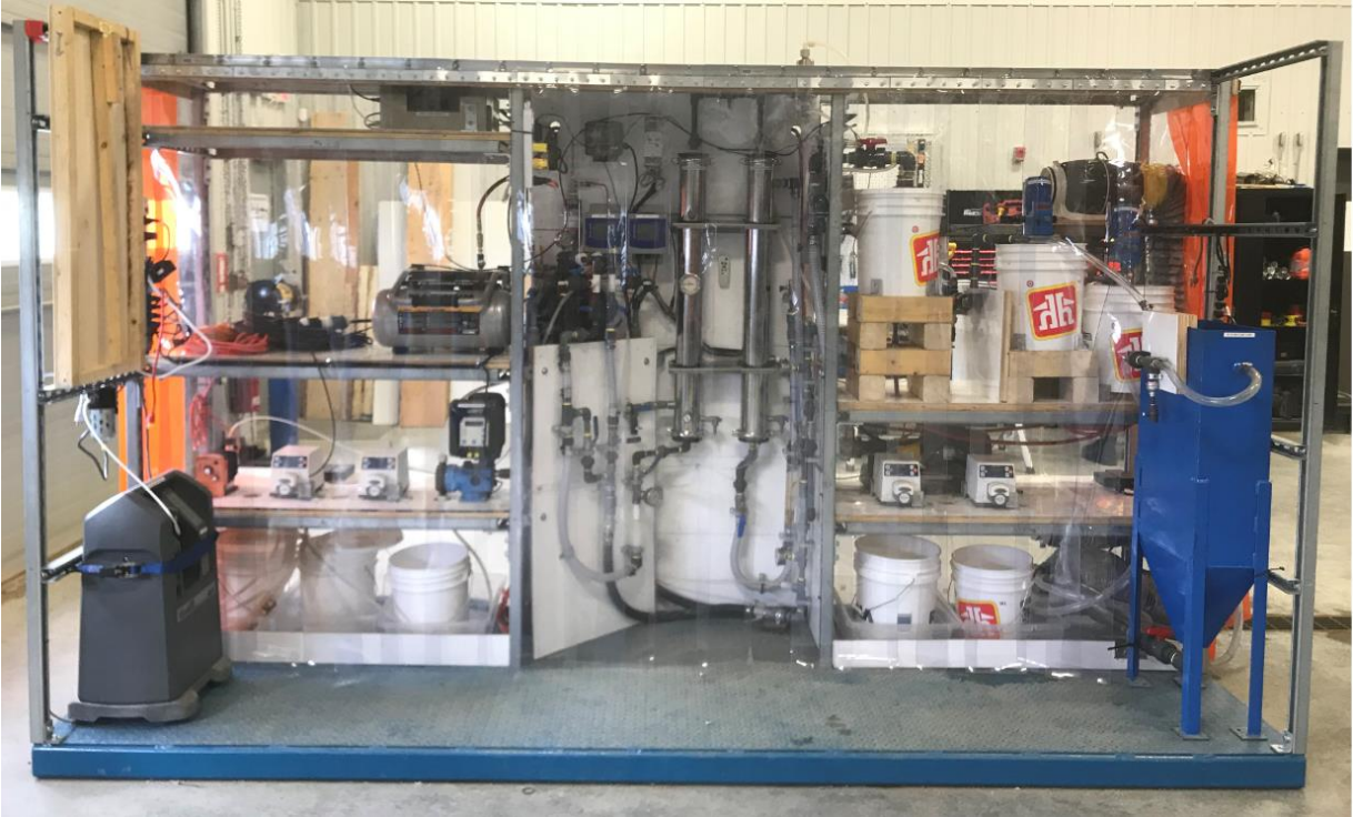
Picture A : Ozone pilot skid
